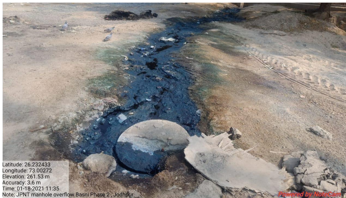
Fig. 1(e): Leakage of CETP Manhole in Basni Phase II industrial area, Jodhpur
