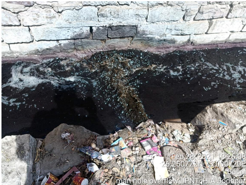
Fig. 1(j): Overflow of Manhole in JPNT, CETP Pipelines in HIA Jodhpur
