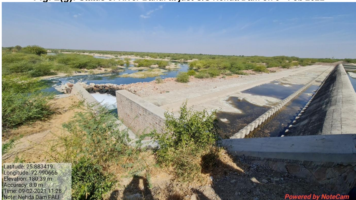
Fig. 2(h): Status of River Bandi at just D/S Nehda Dam on 9 th Feb 2021
