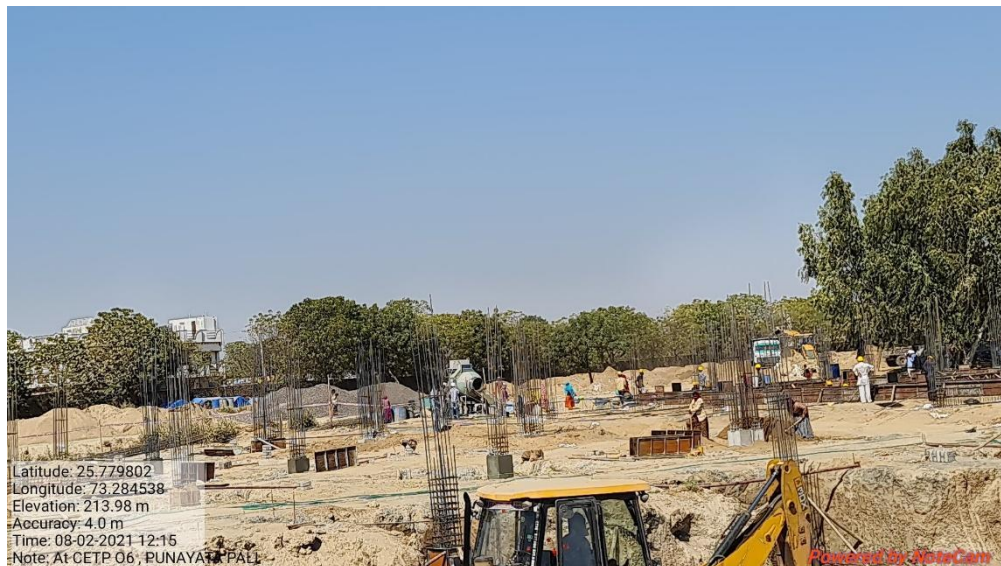
Fig. 2(o): Status of construction of R.O. Plant at CETP 06, Pali
