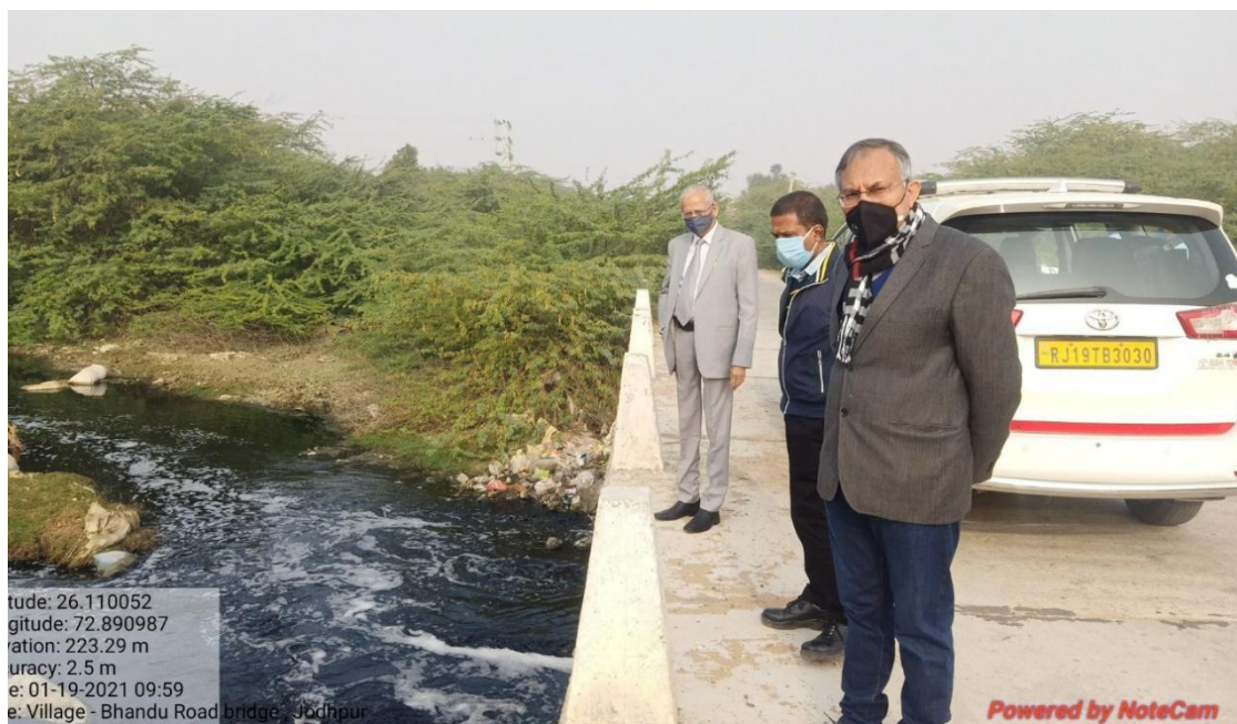
Fig. 1(n): Status of river Jojri at the d/s of culvert site (downstream of Bhandu Village).
