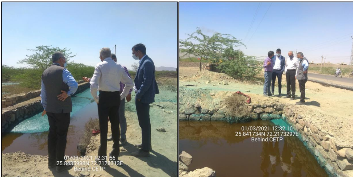
Fig. 3(c): Solar Evaporation Ponds located behind the CETP in Balotra
