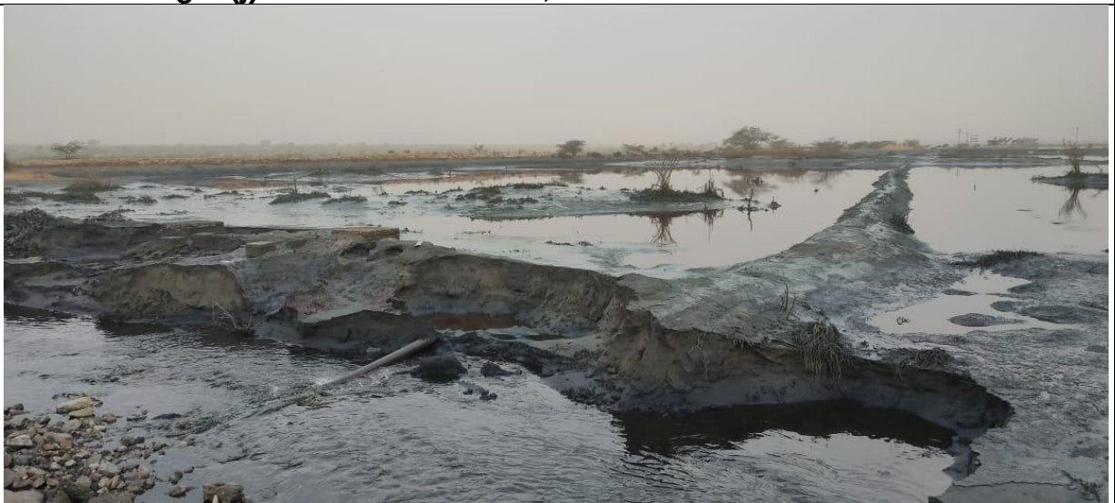
Fig. 3(k): Breach of SEP/HRTS, CETP Balotra on 22 March 2021
