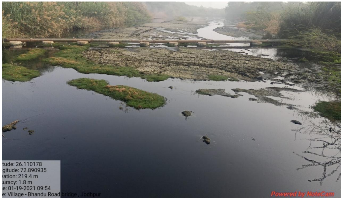
Fig. 1(l): Status of river Jojri at the u/s of culvert site (downstream of Bhandu Village).
