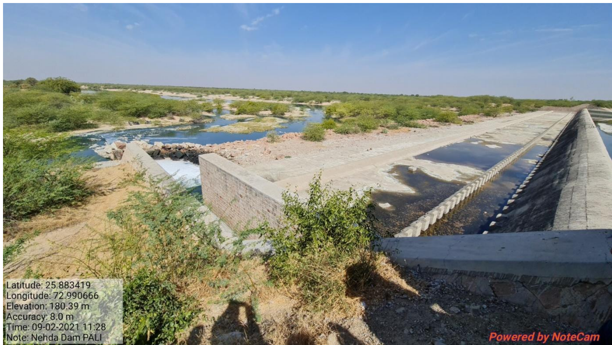
Fig. 2(i): Status of River Bandi at just D/S Nehda Dam on 9 th Feb 2021
