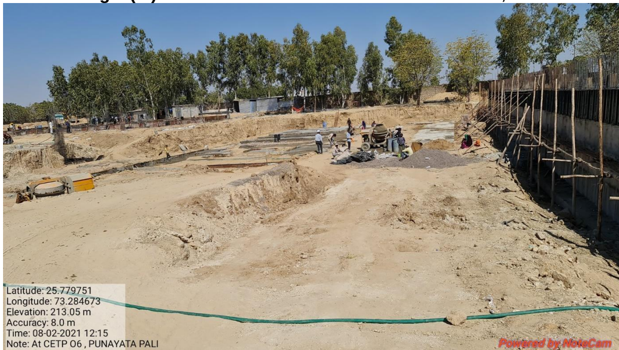
Fig. 2(n): Status of construction of R.O. Plant at CETP 06, Pali
