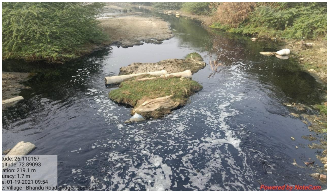
Fig. 1(m): Status of river Jojri at the d/s of culvert site (downstream of Bhandu Village).
