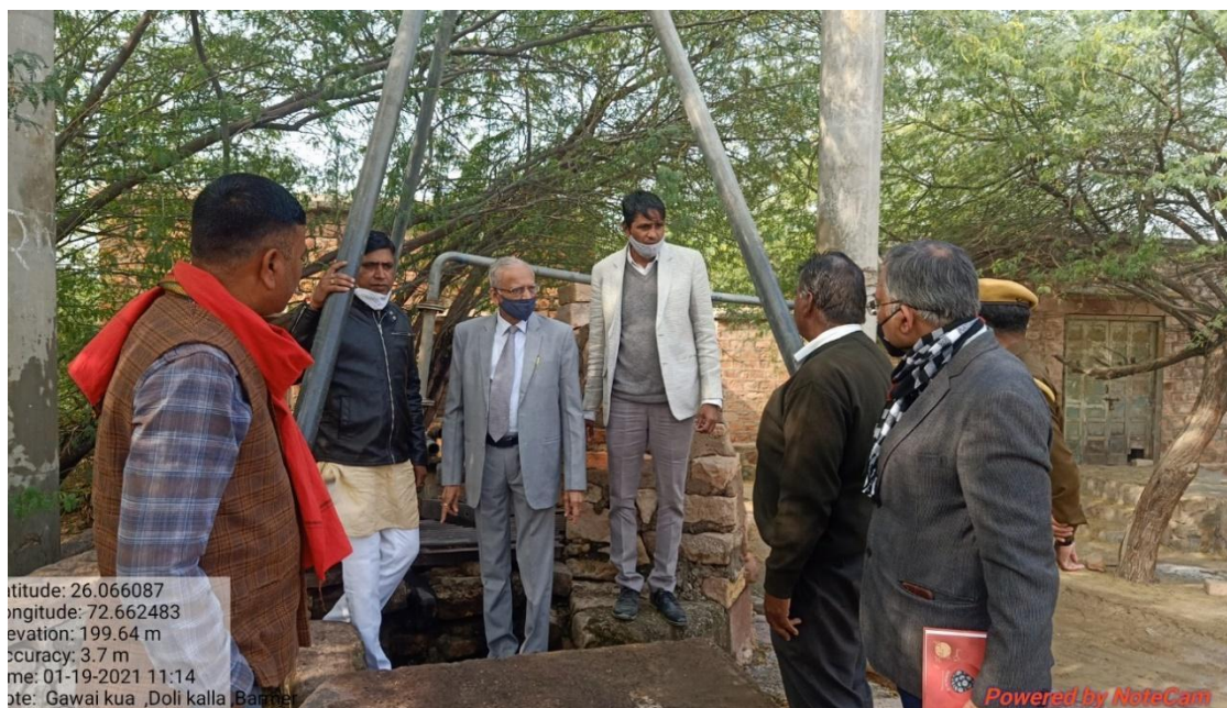
Fig. 1(p): Inspection of defunct well (Pabur Bera, Gawai Kua) which is now not being used due to contamination of water at Doli Village.
