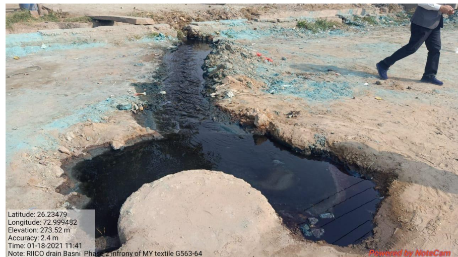
Fig. 1(g): Colored industrial wastewater in Drain due mix of industrial wastewater (Also, blockages in the drain due to rubbish, sand, polythene bags, chemicals, floating materials and solid waste), Jodhpur.
