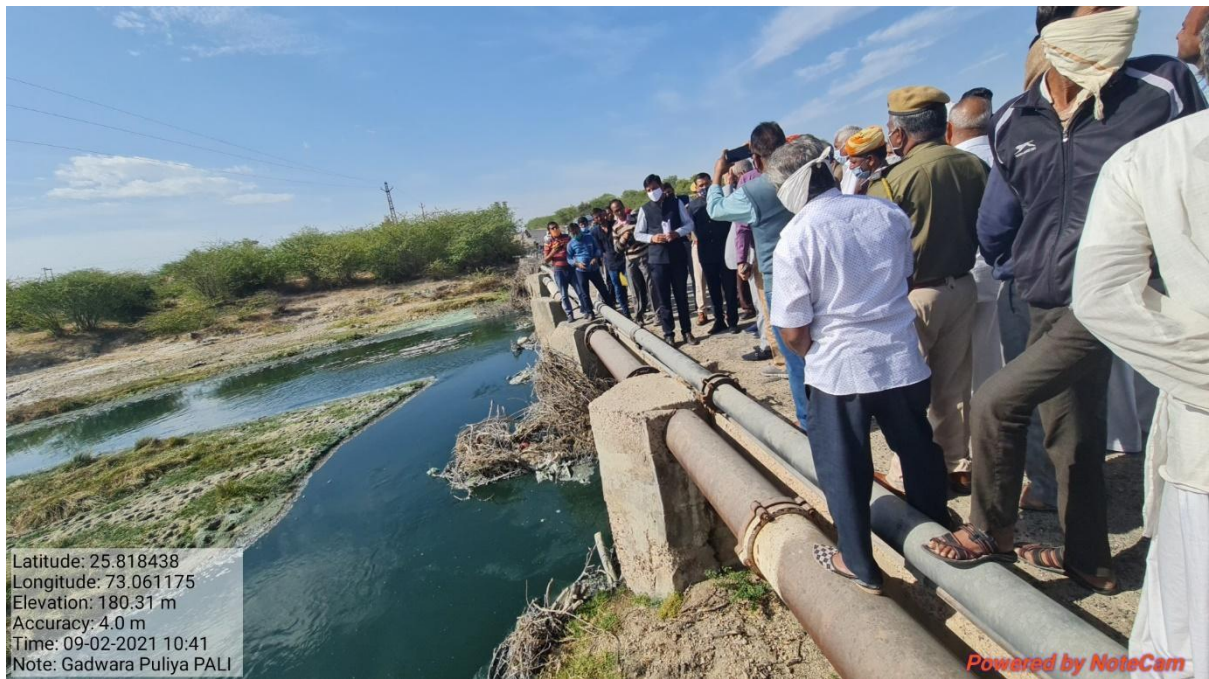
Fig. 2(e): Status of River Bandi at Gadwara Puliya, Pali on 9 th Feb 2021
