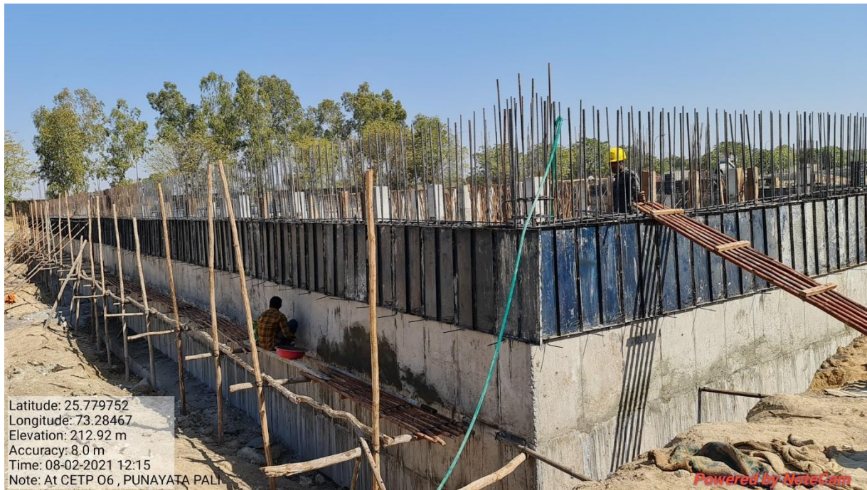
Fig. 2(m): Status of construction of R.O. Plant at CETP 06, Pali
