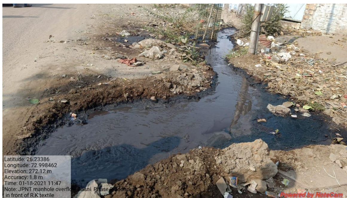
Fig. 1(i): Leakages/overflow of industrial wastewater from a CETP Manhole lead to illicit discharges into Drains, Jodhpur.
