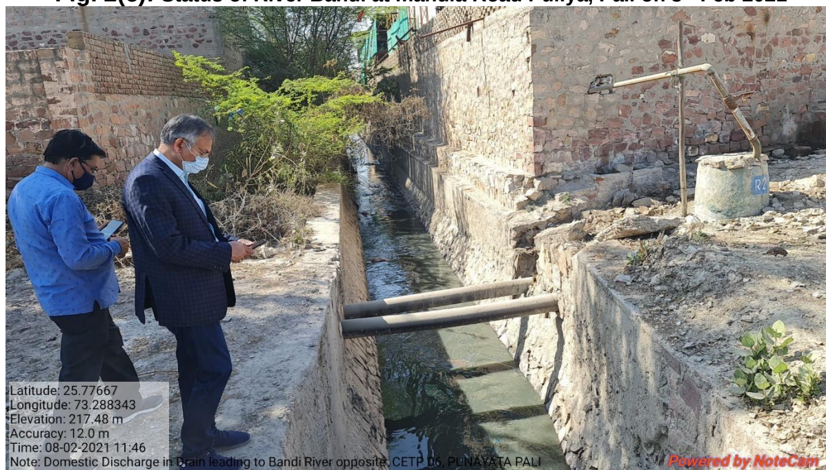
Fig. 2(d): Domestic discharge in a Drain leading to Bandi River opposite to CETP Pali on 8 th Feb 2021
