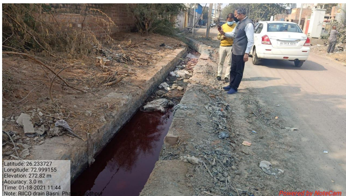
Fig. 1(h): Colored industrial wastewater in Drain (Also, blockages in the drain due to rubbish, sand, polythene bags, leaves, floating materials chemicals and solid waste), Jodhpur.
