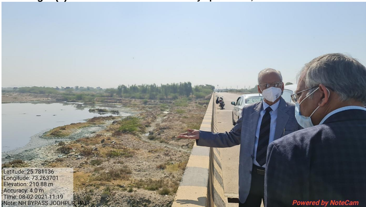
Fig. 2(b): Status of River Bandi at NH Bye pass road, Pali on 8 th Feb 2021
